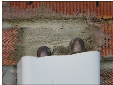
THE CONNECTION OF THE PIPEWORK RUNNING THROUGH THE WALL
