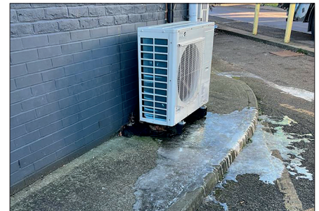
THE HAZARDS WHEN YOUR INSTALL DOES NOT HAVE ADEQUATE SOAK AWAY
