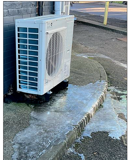
THE HAZARDS WHEN YOUR INSTALL DOES NOT HAVE ADEQUATE CONDENSATE REMOVAL
