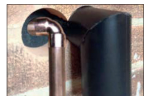
4. Fit the elbow over the copper pipes.
