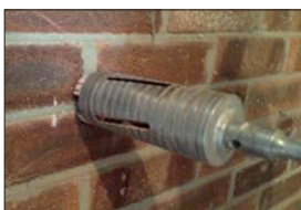
1. Select a 65mm core drill.
