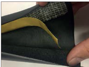
STEP ONE Open the pre-slit insulation.
