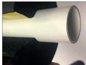
STEP TWO Wrap around the pipe, peel away yellow cover and seal together. Use the adhesive flap to secure.
