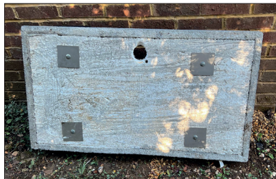
STEP 8 - Attach all 4 base plates to the underside of the slab.
