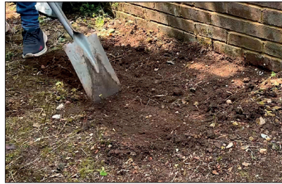
STEP 2 - Prepare the ground.
