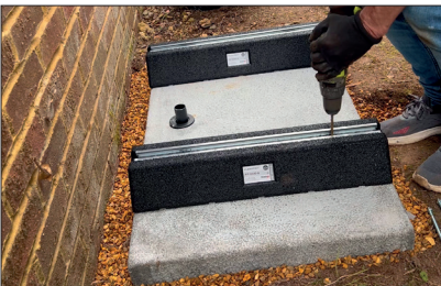
STEP 7 - Place the feet in position, and drill 9mm holes through the feet 50mm from each end.
