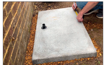
STEP 6 - Measure the slab for the placement of the feet. This needs to match the pitch of the unit.
