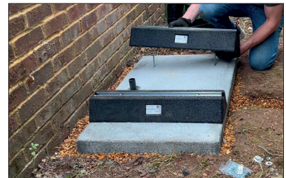
STEP 9 - Place the feet on the threads.
