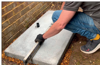
STEP 5 - Ensure that slab is level.
