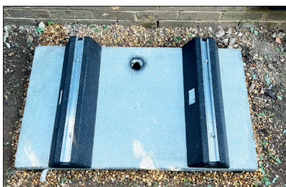
STEP 11 - The Flexi Lite Slab install is complete and ready for the unit
