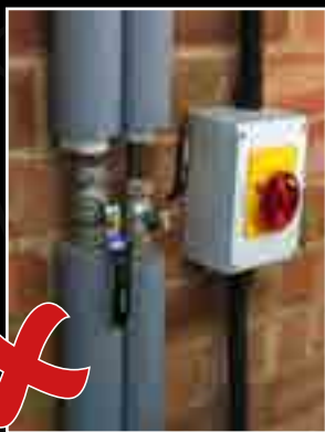
GREY/SILVER INSULATION FOR INTERNAL USE ONLY
