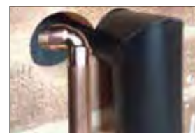
4. FIT THE ELBOW OVER THE COPPER PIPES.
