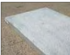
POSITION SLAB IN REQUIRED POSITION
