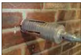
1. SELECT A 65MM CORE DRILL.
