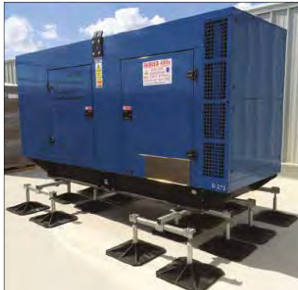
DOUBLE MOUNTING PLATE PART CODE - F-TQ-ADJ-D
