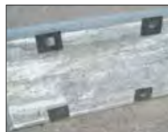
INSERT ALL 4 BASE PLATES THROUGH THE SLAB
