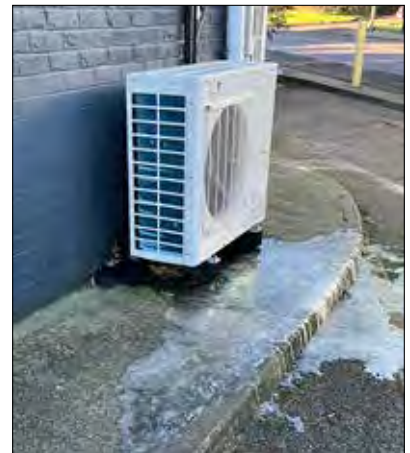
AVOID PROBLEMS RESULTING FROM INCORRECT DISPOSAL OF CONDENSATE
