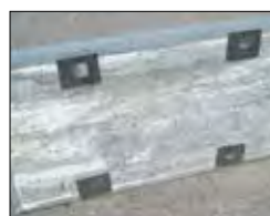
INSERT ALL 4 BASE PLATES THROUGH THE SLAB
