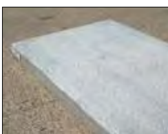
POSITION SLAB IN REQUIRED POSITION
